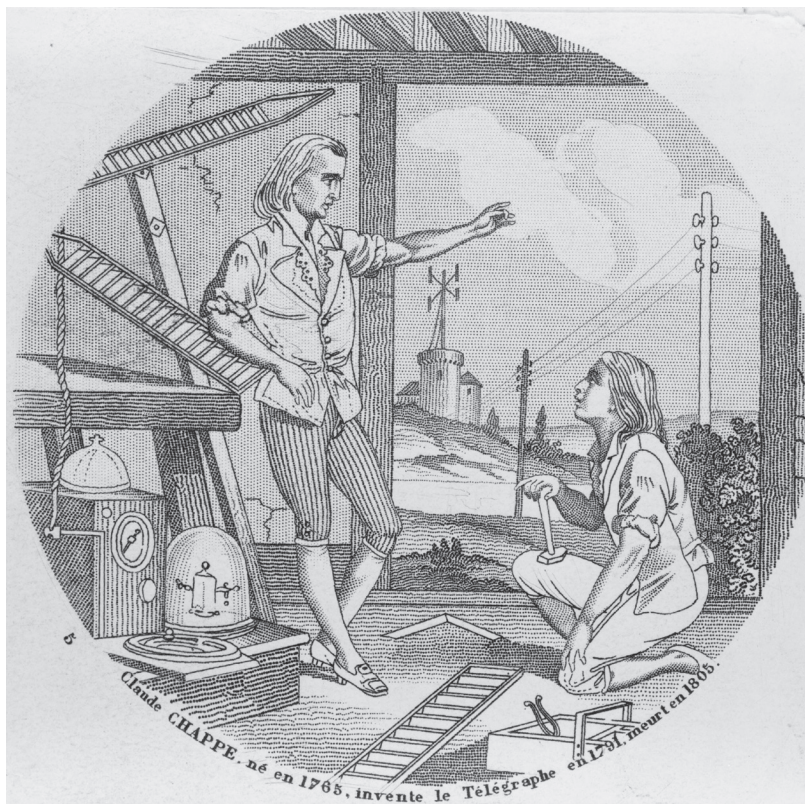
Figure 7.1 First telegraph—The “optical” telegraph was developed by Claude Chappe in France forty years before Samuel Morse began thinking about using electricity for signals over distance. The optical telegraph was too expensive for routine use and could not be used in bad weather. 1805 illustration, Library of Congress.
